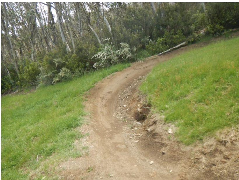
Figure 1 - Existing All Mountain Trail on the Dream Run - with large cuts impeding summer and winter access
